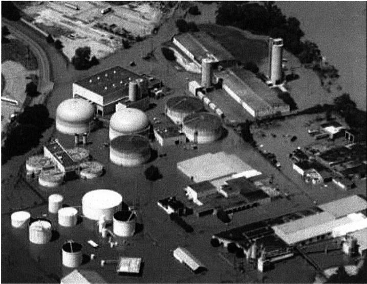
Figure 3.8: Flooding at Biosolids Facility
