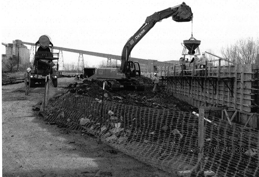
Figure 5.11: Central Biosolids Facility EPS under construction
