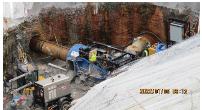
Work progresses at the Davidson Branch facility.
