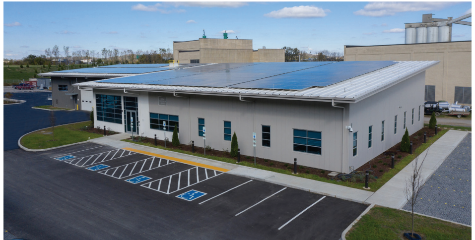
The Central Water Reclamation Facility maintenance building is now complete.
