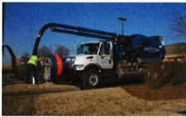
Metro has to clean grease from sewer lines to prevent overflows.
