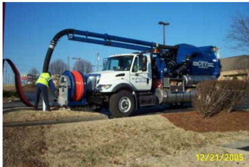
Metro has to clean grease from sewer lines to prevent overflows.
